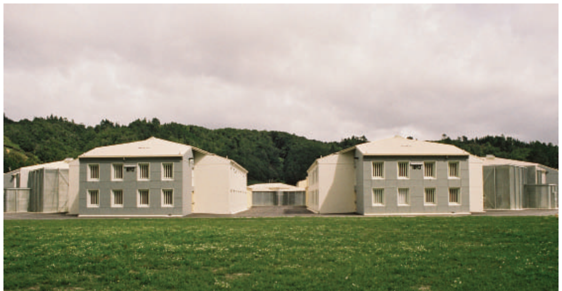
Work by Opus International Consultants Ltd on Rimutaka Prison's new facilities has been entered in the Innovate NZ Awards.
